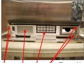
screws Figure 14a HEPA screws metal filter panel
