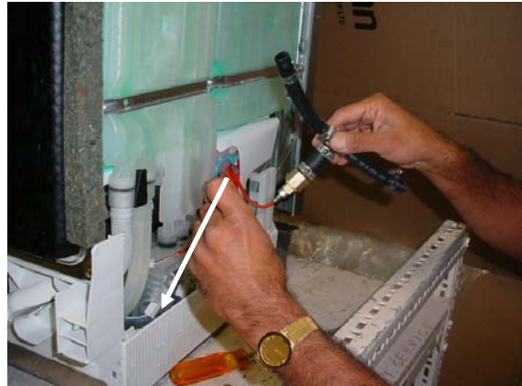
Feed the temperature sensor wire and plug into existing connector.
