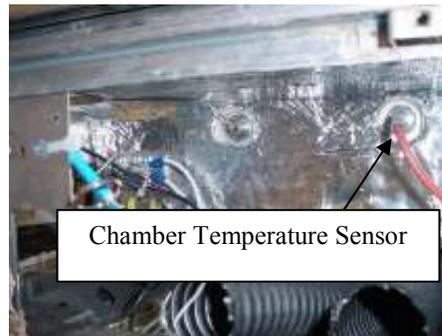
Remove mounting nut from sensor located underneath the filter inside the chamber. Behind the cover below the front door remove the sensor from the chamber and unplug the red wiring. **Chamber Temp. Sensor Part # 22816.12**
